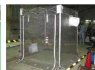
The instant tent for dust scattering prevention For dust scattering prevention at a demolition work site! For noise control
